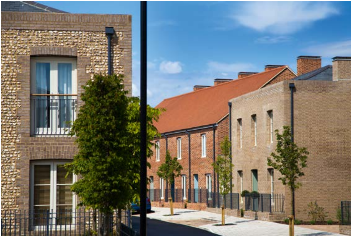
Reworking local materials anchors a building in a place and its history
